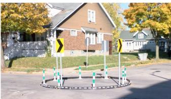
**Milwaukee**, **WI** piloted low-cost, Quick-Build traffic circles .
